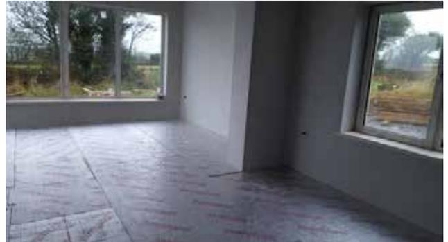
2. **PLASTIC MEMBRANE (P.U. MEMBRANE)** Before placing of underfloor heating pipes a plastic membrane must be installed directly onto the insulation boards, and returned up the walls. This ensures no leakage of the screed and allows the screed to dry consistently throughout. Joints need to be taped and upturns fixed at 150mm above screed levels. (It can be trimmed back after screed is poured.)
