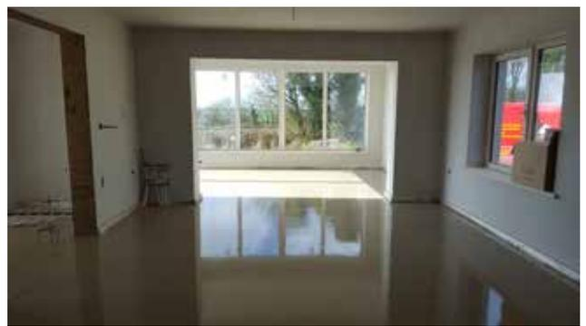
5. **FINISHED FLOOR** Once installed, the screed is left to set, foot traffic can commence after 6- 24 hours (depending on screed type) under normal drying conditions. A moisture test is advised prior to laying floor coverings.
